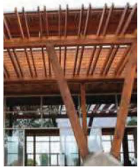
Heavy timber construction
