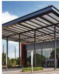
Structural metal framing/steel framing
