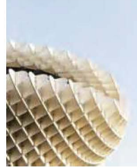
Exposed glulam construction
