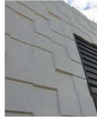
Pre-cast concrete panels
