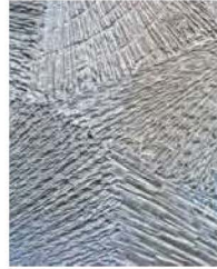
Stamped concrete/ Concrete finishing
