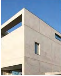
Cast in place concrete
