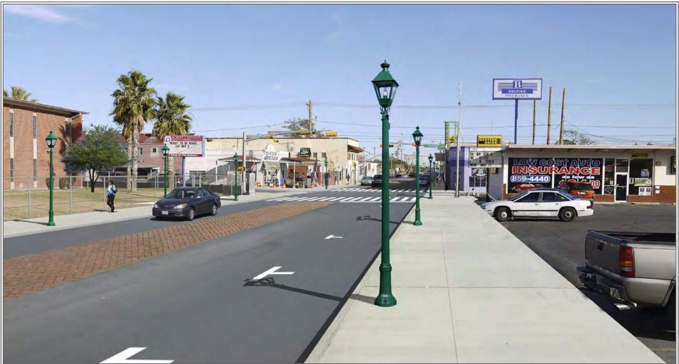
Step 1: Public improvements can be made that will enhance the pedestrian environment. Travel lanes in this section of Alameda Avenue should likely be reduced to one lane in each direction with a central left turn lane. This creates enough space within the right-of-way to add on-street parking to one side of the street. By widening the sidewalk, introducing pedestrian scaled lighting, and on-street parking, pedestrians begin to have a more comfortable, protected setting.
