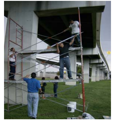
Just hard work getting the 30-foot high columns prepared!
