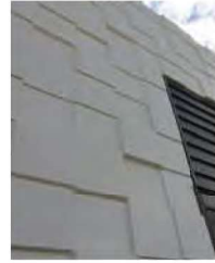
Pre-cast concrete panels
