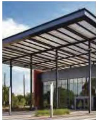
Structural metal framing/steel framing
