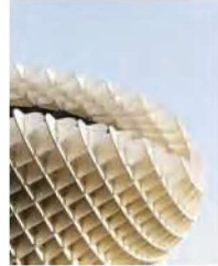
Exposed glulam construction
