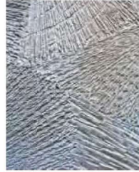
Stamped concrete/ Concrete finishing
