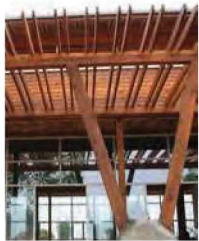
Heavy timber construction
