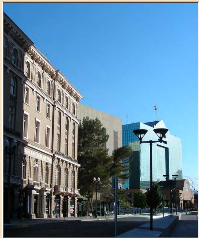
The El Paso County Courthouse is unquestionably “of its time” and distinct from its setting in historic Downtown El Paso, however the utility of glass curtain wall construction in El Paso’s desert setting is inconsistent with climate-sensitive vernacular wisdom.
