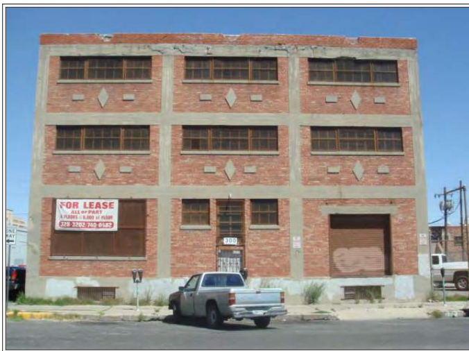
Trost & Trost warehouse building before rehabilitation
