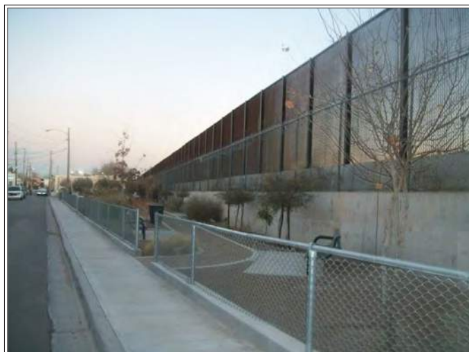
International fence along the United States/Mexico border in the historic Chihuahuita neighborhood.
