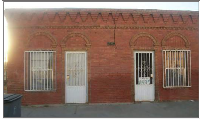
Windshield surveys and photographic surveys conducted by community groups can serve as a first step towards identifying and protecting historic resources, such as this duplex in Chamizal.
