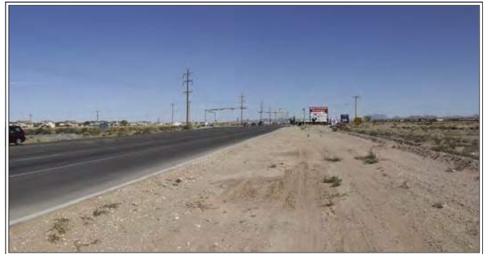
Existing conditions on Zaragoza Road include high speed travel lanes and wide dirt medians making vehicular transportation the only option.
