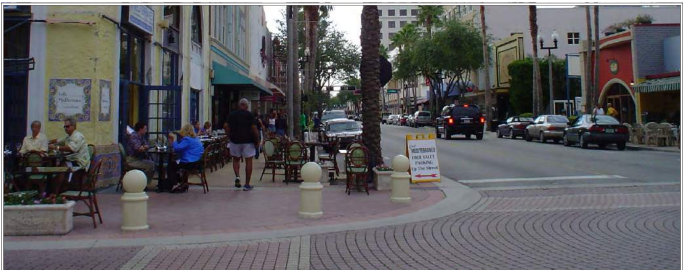
A curbless intersection with bollards allows for pedestrian confidence while accommodating the turning radius of emergency response vehicles.
