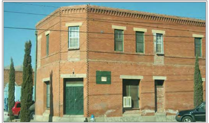
Historic mixed-use building in Segundo Barrio. To date, community opinion has been against historic preservation, because residents fear it will lead to gentrification.
