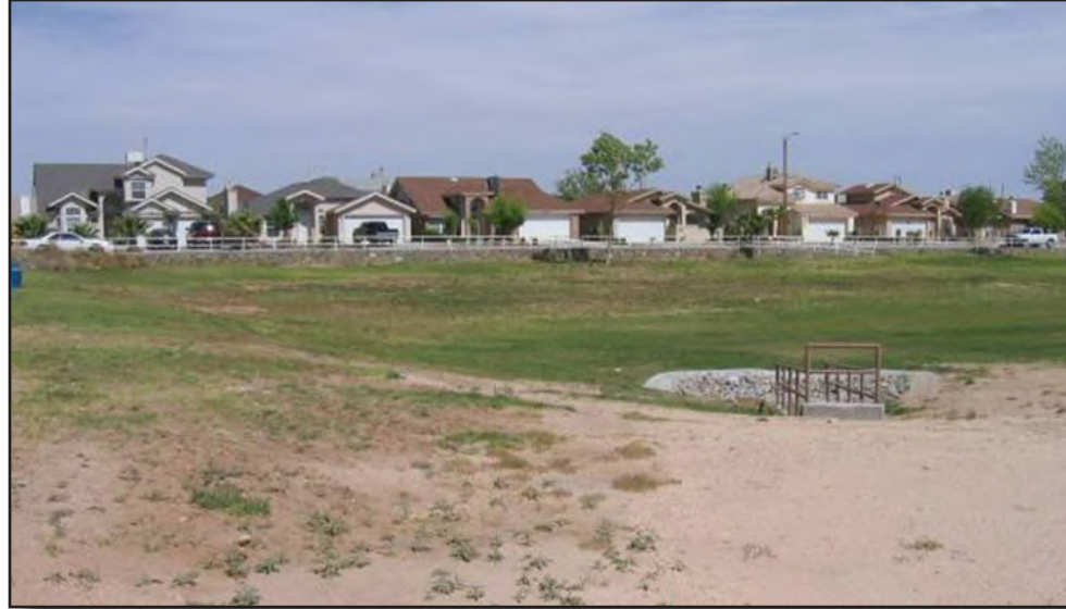
Continue to convert detention areas into dual use park/ponds. Photo by Halff Associates
