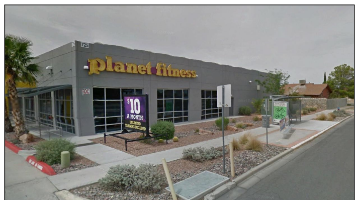
Windows that are mirrored, have opaque graphics, or a visible light transmittance lower than 60% cannot be counted toward the transparent façade area.
