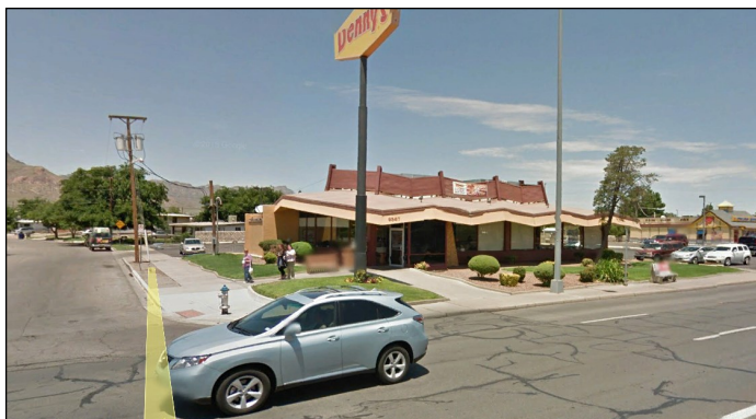
This restaurant is placed at the corner of the lot, with entrances facing the street. Parking is provided on-site, but it is located to the site and rear of the lot. The building is the most prominent feature of the lot, and its entrances, windows and landscaping contribute to the streetscape.
