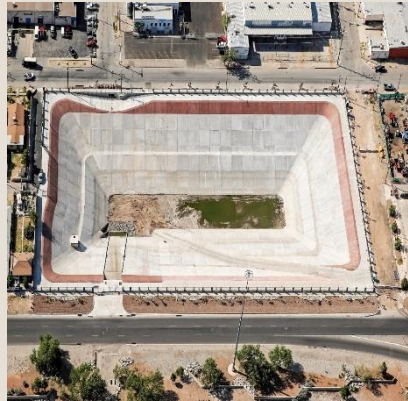
Gateway East Pond added 27 Million Gallons of storage $5.7M
