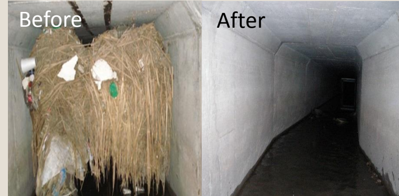
Dallas Conduit Clearing of Utilities $1.4M
