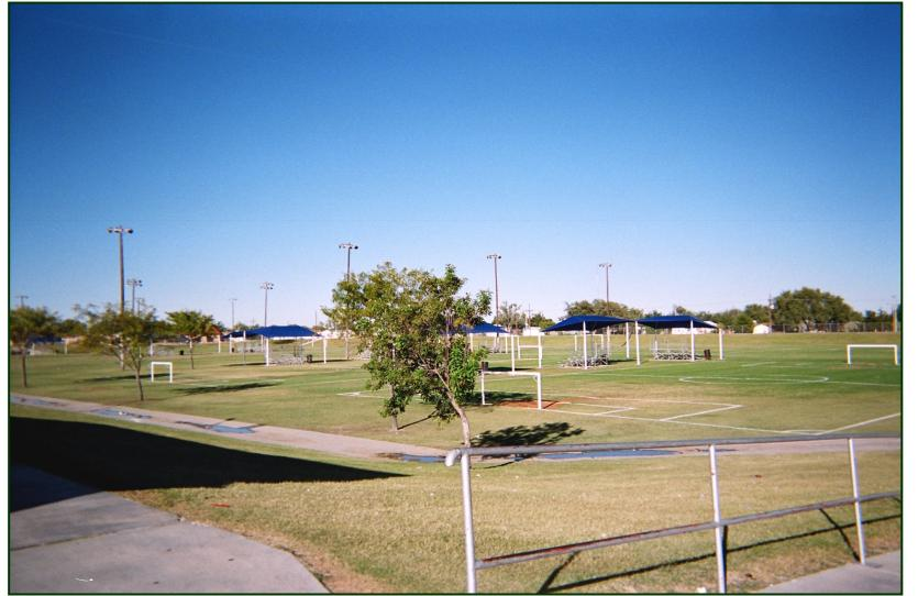
**Hobbs, New Mexico** – Soccer Complex built into a regional detention pond. Note pilot channels for periodic flow (also used as sidewalks), raised structures, and flood outflow structure. The entire area is contained by a fence for closure during flood events. Restrooms and concession facilities are located along the top of the adjacent levee. Stairs and ramps provide access from parking and surrounding prior backs and surrounding prior backs are set of the adjacent leves. neighborhoods.
