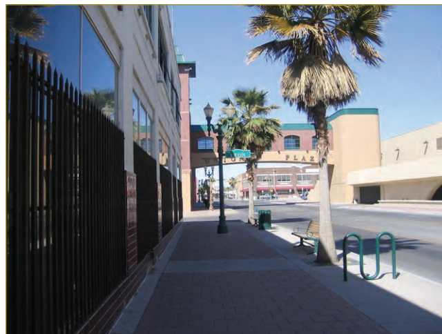
Top Overland Street Apartments
