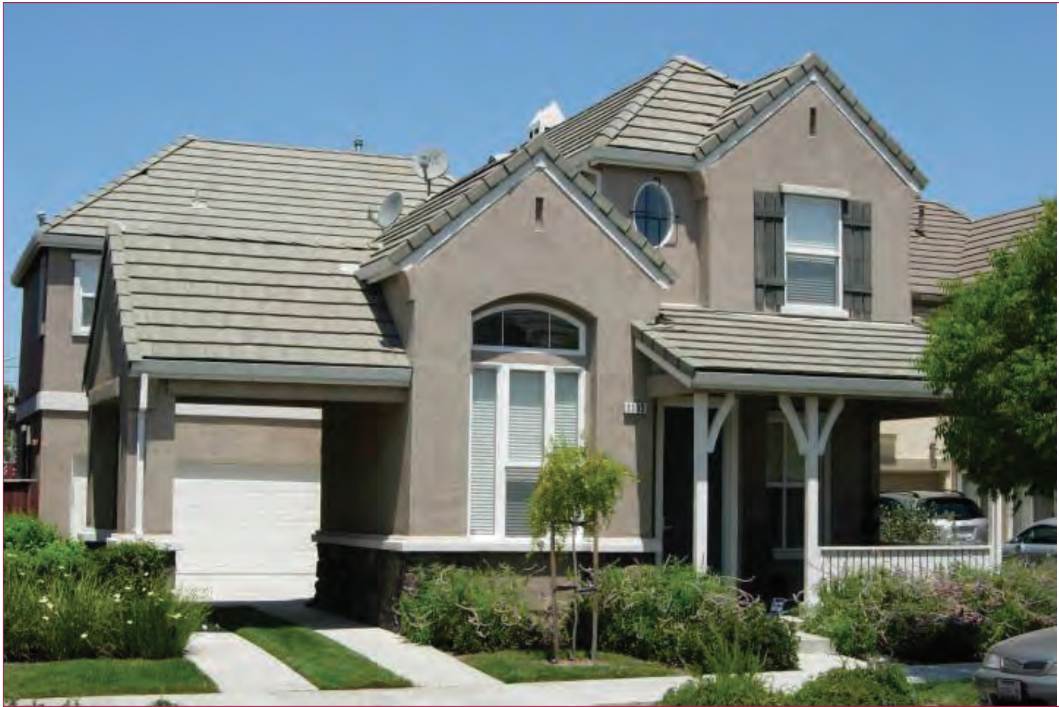
Single Family residence with garage behind the main house
