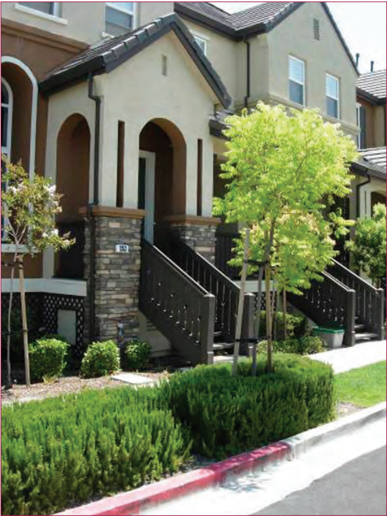
Townhomes with main level raised atop a partially sunken parking level
