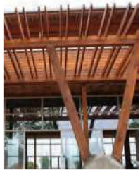
Heavy timber construction
