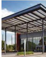
Structural metal framing/steel framing
