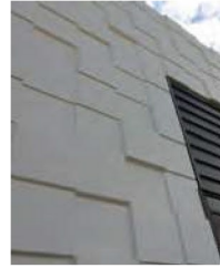
Pre-cast concrete panels
