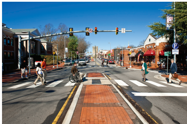
Figure 58. An example of a complete street from the Walk.Bike.NC complete streets program in Raleigh, North Carolina
