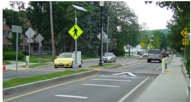
Figure C24. A raised crosswalk doubles as a speed table to reduce motor vehicle speeds.
