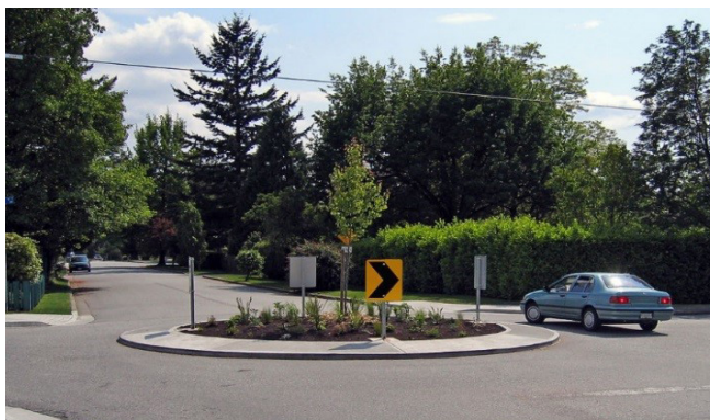
Figure C25. Traffic circles have proven to be effective intersection treatments for bicycle boulevards.
