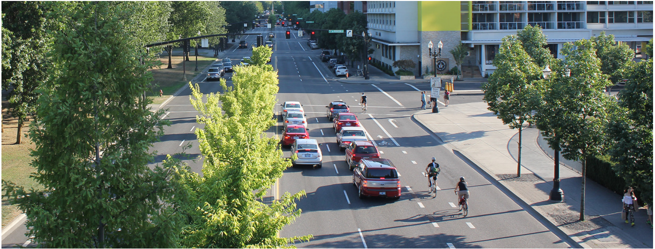
Figure C7. Drivers wishing to enter the right turn lane must transition across the bicycle lane in advance of the turn.
