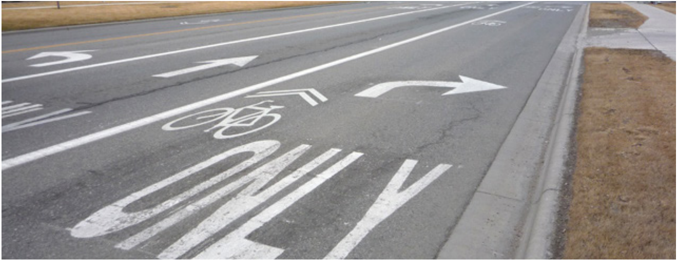
Figure C9. Shared lane markings and signs indicate that bicyclists should ride on the left side of this right turn only lane.
