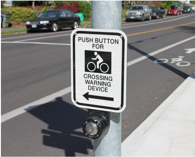
Figure C16. Bicycle push button actuators are positioned to allow bicycle riders in roadway to stop traffic on busy cross-streets.
