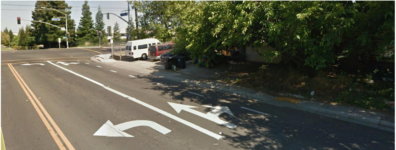
Figure C6. The dashed bike lane line on Lincoln Village Dr signals to drivers that they should enter the bike lane to make their right turn.
