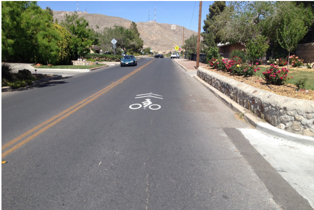
Figure 39. Example of an existing marked shared roadway along Kerbey
