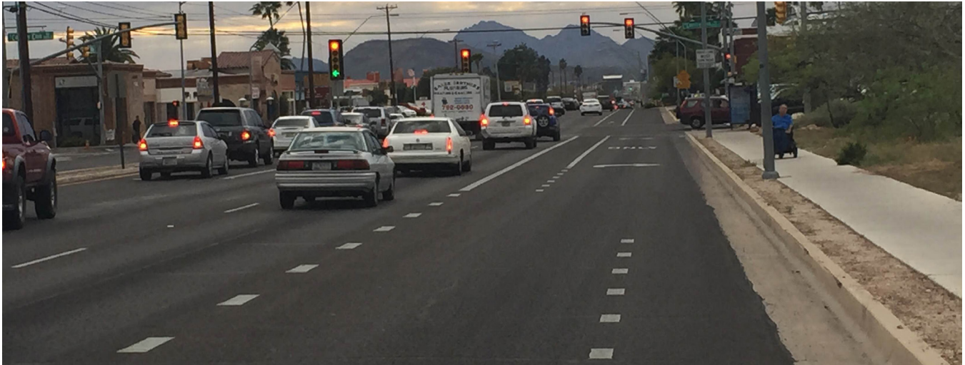
Figure C8. When a through travel lane is “dropped” and transitions directly into a right turn only lane, only confident adult riders can be expected to transition across the lane into the through bike lane. Designers should provide adequate room for bicyclists to take advantage of gaps in traffic, and not prescribe a defined travel path across the turn lane.
