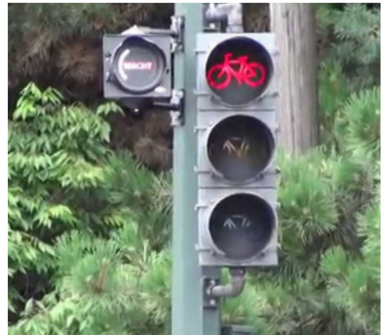
Figure C21. A countdown signal beside the bicycle signal head informs waiting bicyclists of the time remaining until a green signal.
