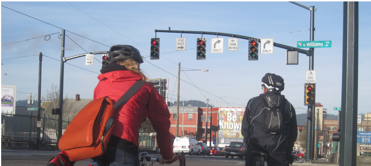
Figure C20. A bike lane adjacent to double right turn lanes normally requires a stressful, difficult maneuver to avoid conflict. With a bicycle signal, conflict is regulated and the conditions are improved.
