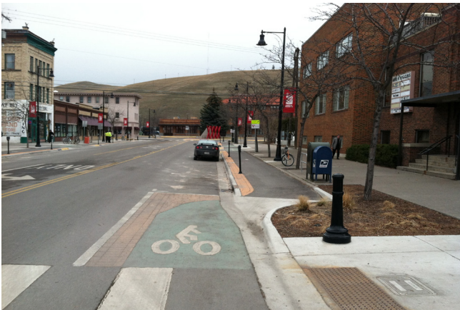
Figure 49. Example of a protected bike lane in Missoula, Montana
