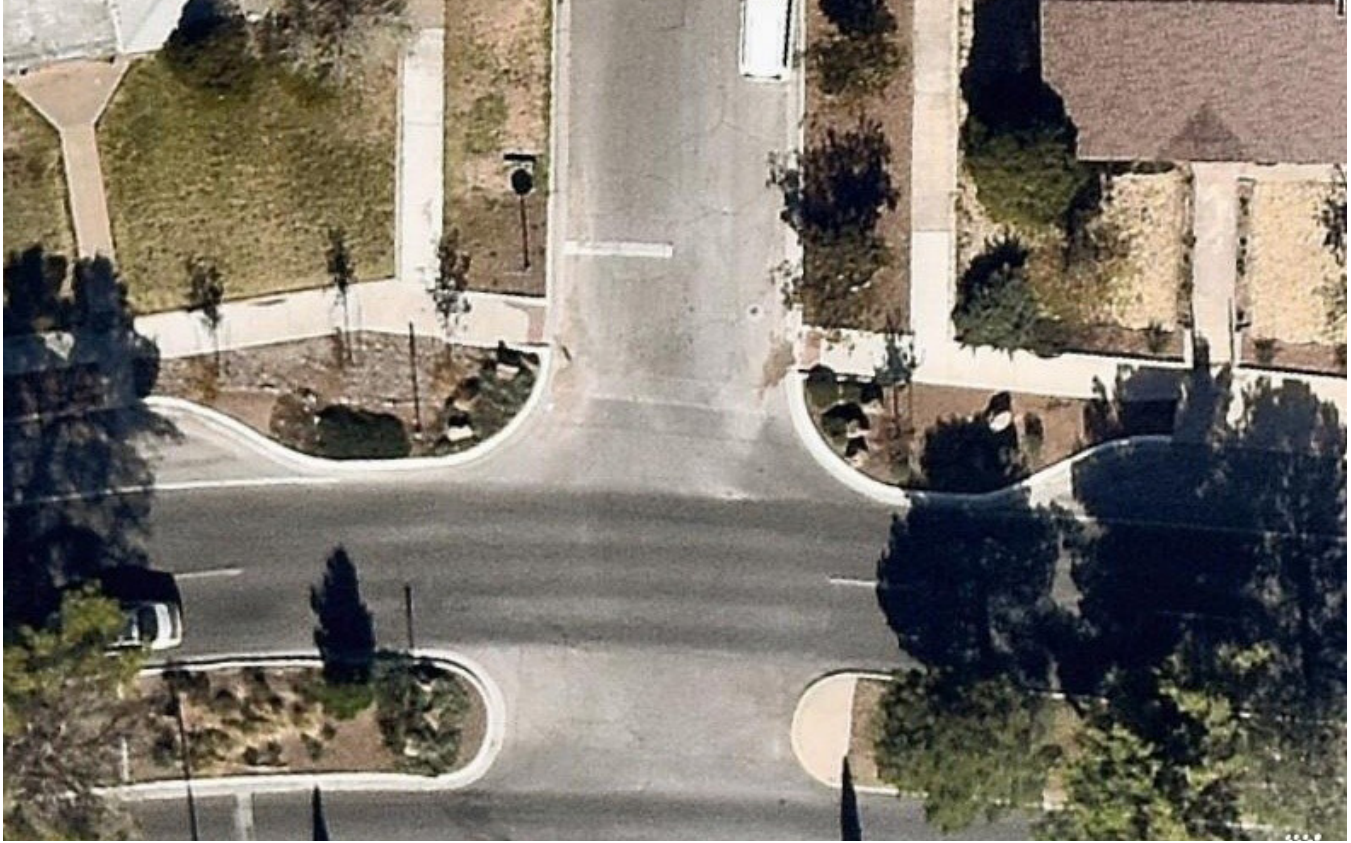
Figure 9. Curb extensions used as a traffic-calming device on Pennsylvania Place and Trowbridge Drive (Source: ©2016 Nearmap.com)
